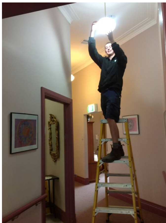
Aaron our electrician modifying Caladenia's lights
